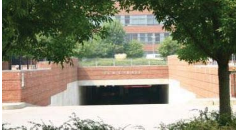
Figure 44: Tunnel to the main Entrance/Exit of the CCM Garage
