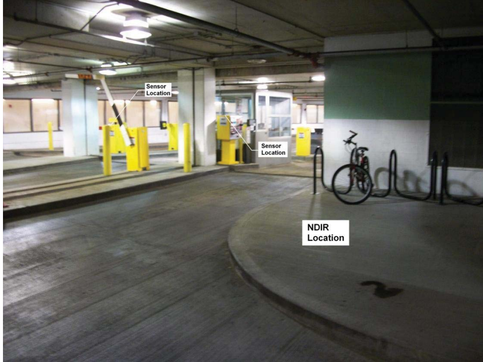
Figure 45: CCM Main Entrance/Exit
